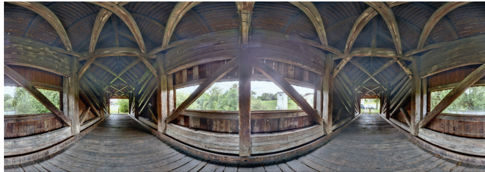
Photo-realistic scan of a old bridge with the HDR Cam
